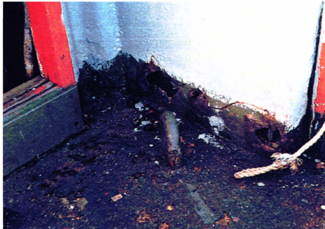
Photograph 1 Corroded accommodation house side structure
