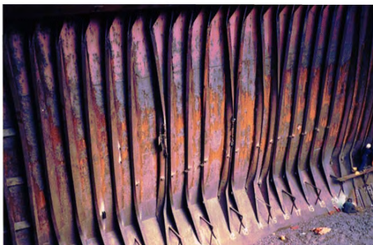
Photograph 1 Collapsed side shell frames (See Example 4)
