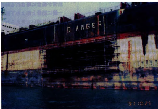
Photograph 2 Missing side shell structure (See Examples 4 and 5)
